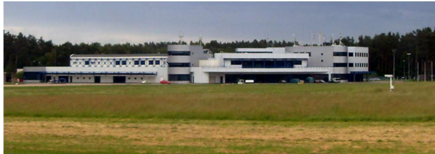
Figure 31. General view of the Goleniów Airport [31].
